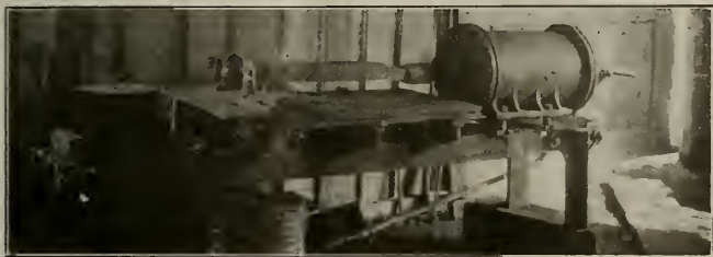
PRESS FOR MAKING BRAKE HANGERS, RECLAMATION PLANT DEPARTMENT, VIRGINIAN RAILROAD.
